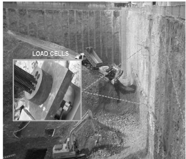
Figure 6. Load cells and instrumented pile.
