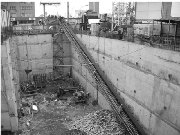
Figure 14. Ground anchors execution.
