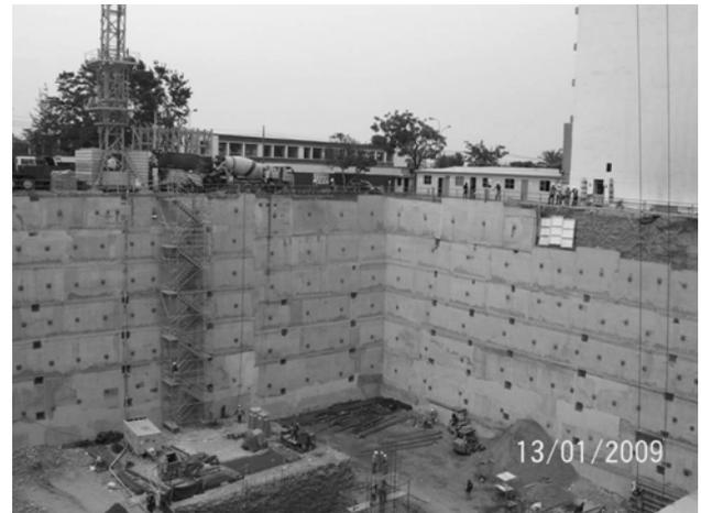
Figure 15. Republica Building with 28 m depth excavation.
