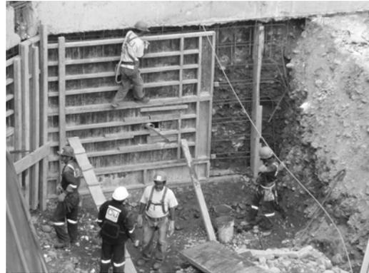
Figure 10. Formwork positioning
