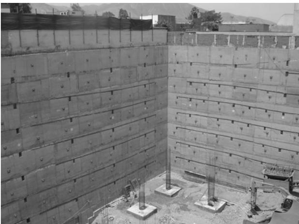
Figure 9. Anchored wall in Lima.
