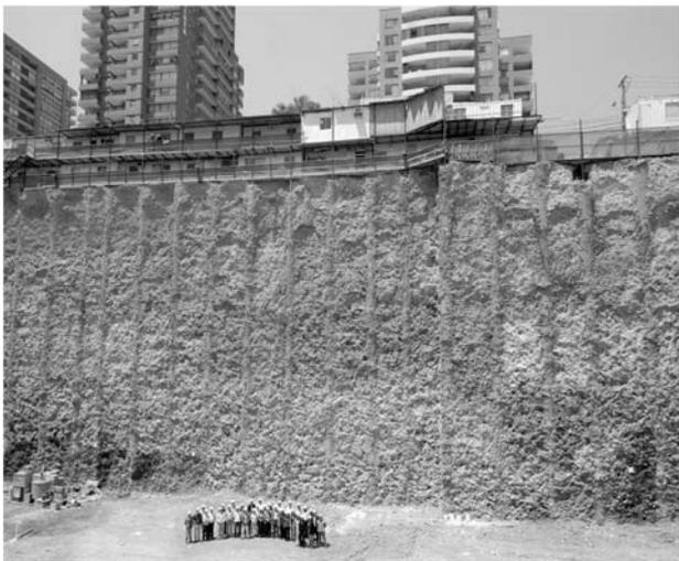
Figure 1. Deep excavation of 28 meters in Santiago.
